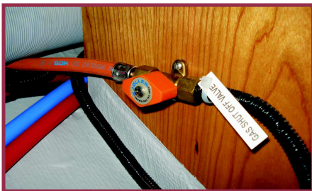
1. Installation valve under the cooker
