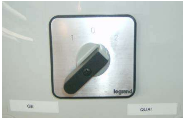
Generator (GE) / Shore power (QUAI) selector switch
