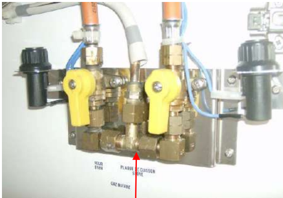
Gas shut off valves under sink
