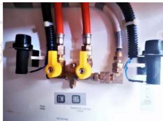
Propane shut-off valves
