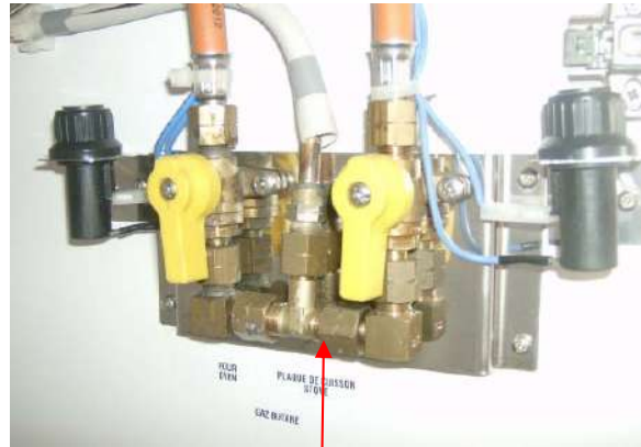
Gas shut off valves under sink
