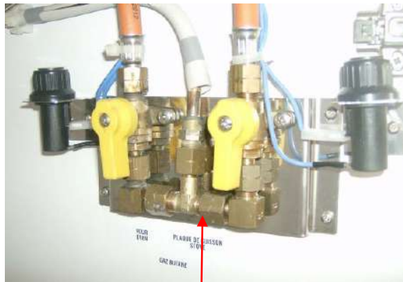
Gas shut off valves under sink
