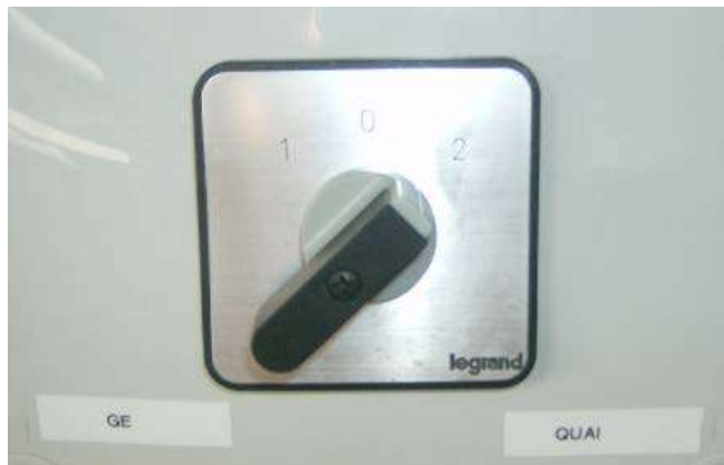
Generator (GE) / Shore power (QUAI) selector switch
