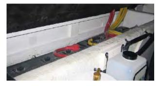
BATTERY CHARGERS: Located above the Batteries on each side of the engine room are the battery Charges. The chargers have an AC input from your 120 volt supply, and a 24 volt output.
