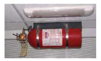
The photo above shows the FM 200 Unit in the Engine Room. The **Automatic Fire Extinguisher System (AFE)** is designed for use in enclosed compartments that are not normally occupied by passengers and are not normally subject to weather or water exposure. The automatic fire extinguisher is designed to extinguish Class B fires (flammable liquids) and Class C fires (electrical), which would be the type that would normally occur within the confined area of the engine/generator compartment.
