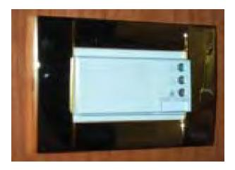
The CO Monitor System has three indicator lights (GREEN, YELLOW, and RED) which illuminate on the control panel. When the monitor is installed, these indicator lights will light up simultaneously for about 1 second, followed by a short buzzing signal, and after which, they will go OFF. Following this process, the three indicator lights will illuminate according to the code of the monitor.
