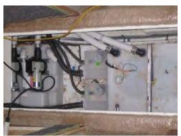
The Shower Sump Pump System operates on 24V DC electrical power. The fuses for the Shower Sump Pumps are behind the DC Electrical Panel in the Salon. Refer to the Electrical Pages of this section of this Owner's Manual for the location of the fuses.
