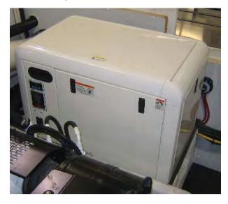
Before the AC Power goes to the AC Main Panel in the Salon, it goes through a breaker on the face of the generator.
