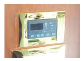
Each air conditioning unit will operate in a "**Dehumidification**" mode upon demand and is controlled by the "Elite Control".
