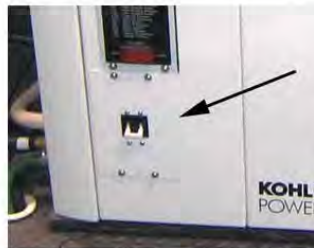
Breaker: Located on bottom of the Generator.
