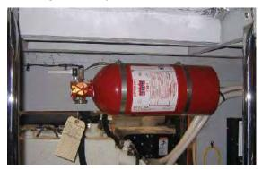
The Automatic Fire Extinguisher System (AFE) is designed for use in enclosed compartments that are not normally occupied by passengers and are not normally subject to weather or water exposure. The automatic fire extinguisher is designed to extinguish Class B fires (flammable liquids) and Class C fires (electrical), which would be the type that would normally occur within the confined area of the engine/generator compartment.
