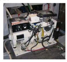
There is a breaker for the generator power above the generator. The generator creates the AC power which goes through the breaker on top of the generator, the ac power then goes to the generator portion of the slide switch on the AC Panel.
