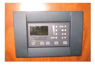
Each air conditioning unit will operate in a "**Dehumidification**" mode upon demand and is controlled by the "Elite Control". Refer to the *Marine Air Systems* Operation and Maintenance Manual for a complete description and instruction in the operation of this mode.
