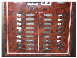
**Converter:** Supplies power to the converter, which converts AC power to DC power.
