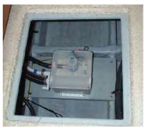
The **Shower Sump Pump System** operates on DC electrical power, controlled by a breaker switch located on the AC/DC electrical Panel (Refer to the Electrical Pages of this section of this Owner's Manual for the location of the switches).
