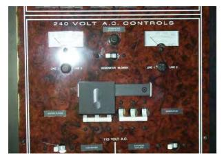
The AC electrical system is supplied with 240 volts of power upon entry to the main electrical distribution panel, which then is separated into two (2) legs of 120 volts each.
