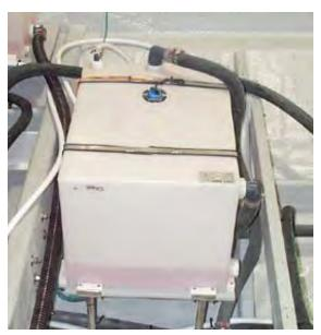
The Waste Tank is equipped with an electronic Waste Level Gauge, which monitors the volume of waste in the tank for your convenience in determining when pumpout is required
