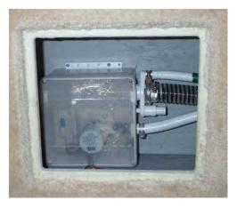
The Forward Shower Sump pump is accessed through the hatch in the deck of the Galley. The photo below shows the Forward Shower Sump Pump.
