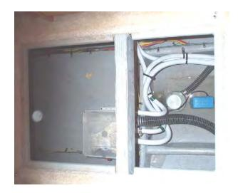
The **Shower Sump Pump System** operates on DC electrical power. There are fuses for these pumps located behind the AC/DC Panel.
