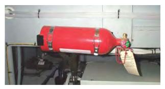
The Automatic Fire Extinguisher System (AFE) is designed for use in enclosed compartments that are not normally occupied by passengers and are not normally subject to weather or water exposure. The automatic fire extinguisher is designed to extinguish Class B fires (flammable liquids) and Class C fires (electrical), which would be the type that would normally occur within the confined area of the engine/generator compartment.
