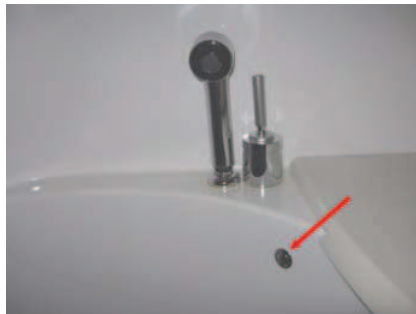
Control Draining pump for shower
