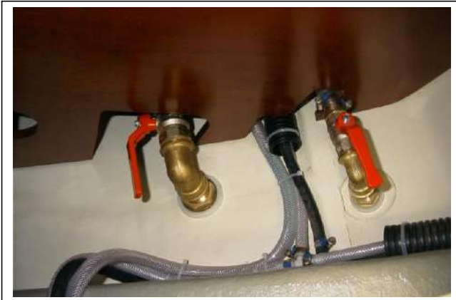
ABB.: RAPID SHUT OFF VALVE – WET AREA
