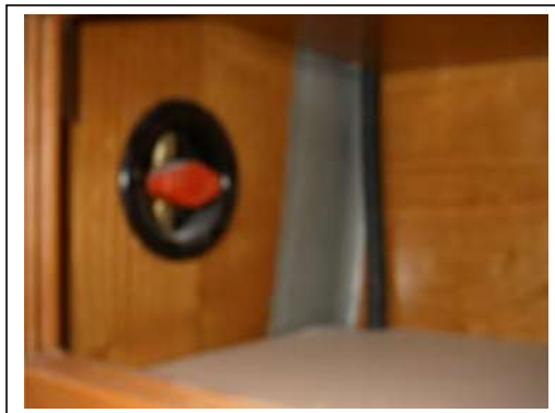
ABB: GAS SHUT-OFF VALVE
