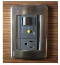
The GFCI receptacles are identified by Test and Reset buttons located between the receptacles' two outlets.
