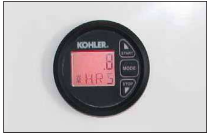
Cabin Generator Control Switch & Monitor
