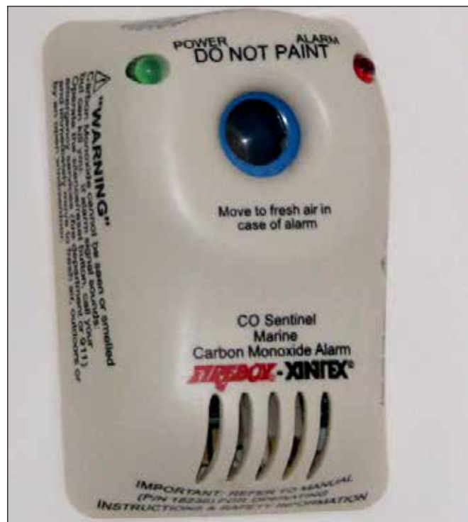
Typical Carbon Monoxide Detector & Alarm
