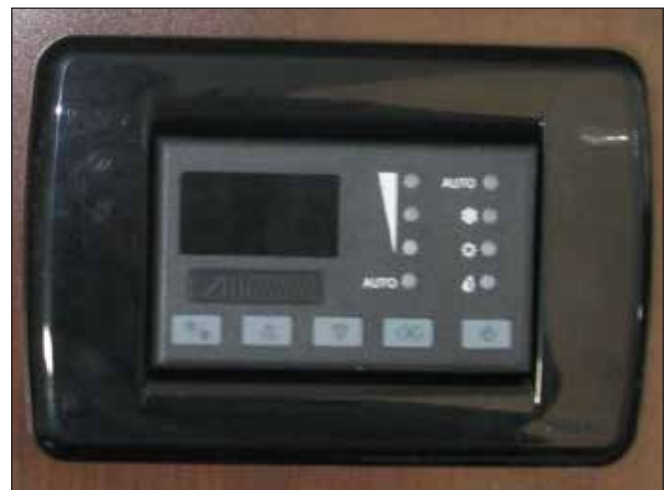
Air Conditioner Control Panel
