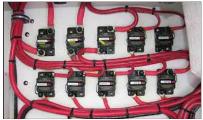
Heavy Duty Main Circuit Breakers
