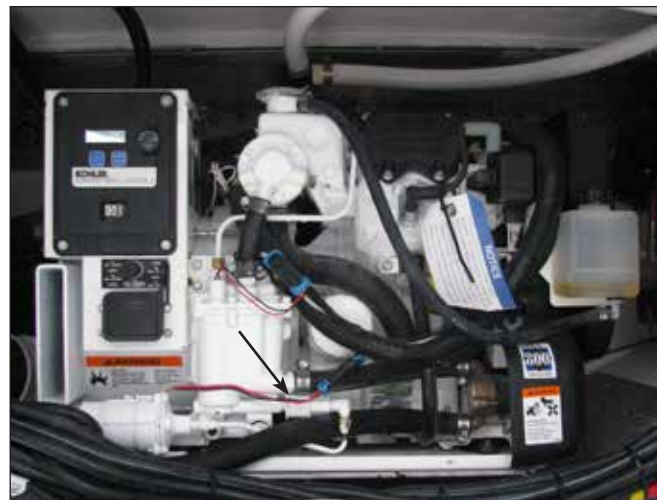
Generator In-Line Fuel Filter
