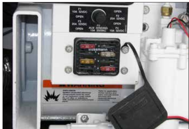
Typical Generator Fuse Panel
