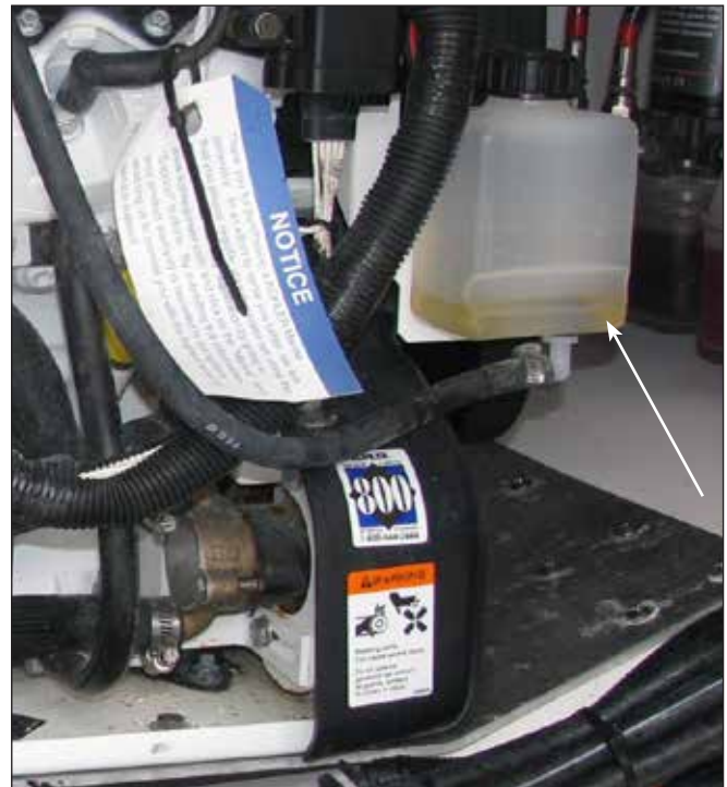
Generator Coolant Recovery Tank
