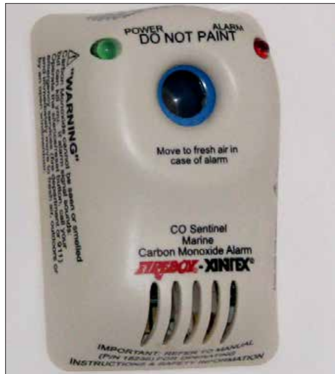
Typical Carbon Monoxide Detector & Alarm
