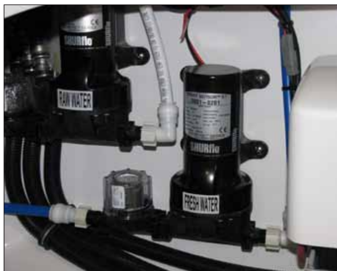
Fresh Water Pump and Strainer
