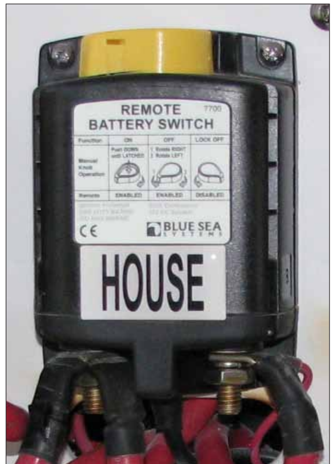
Typical Remote Battery Switch
