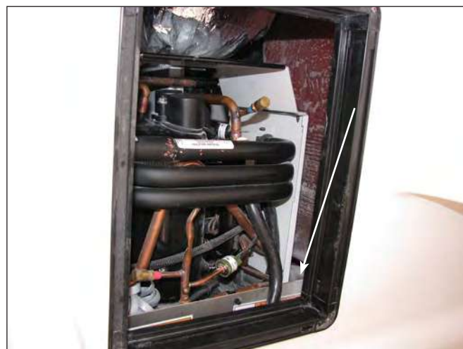
Typical Air Conditioning Condensation Pan
