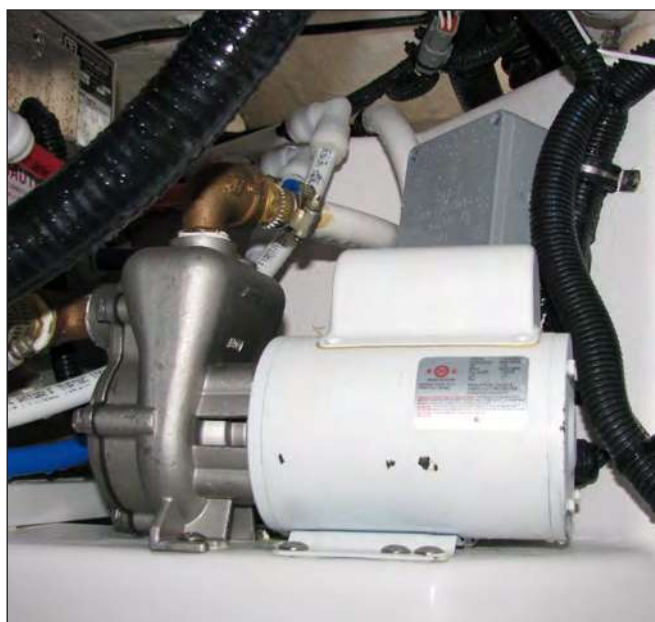
Air Conditioner Seawater Pump
