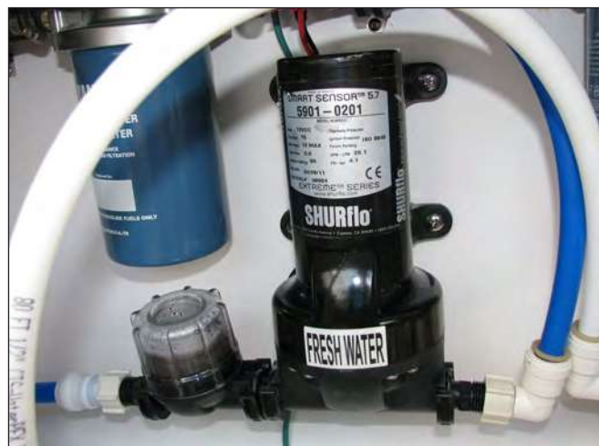
Typical Fresh Water Pump and Strainer
