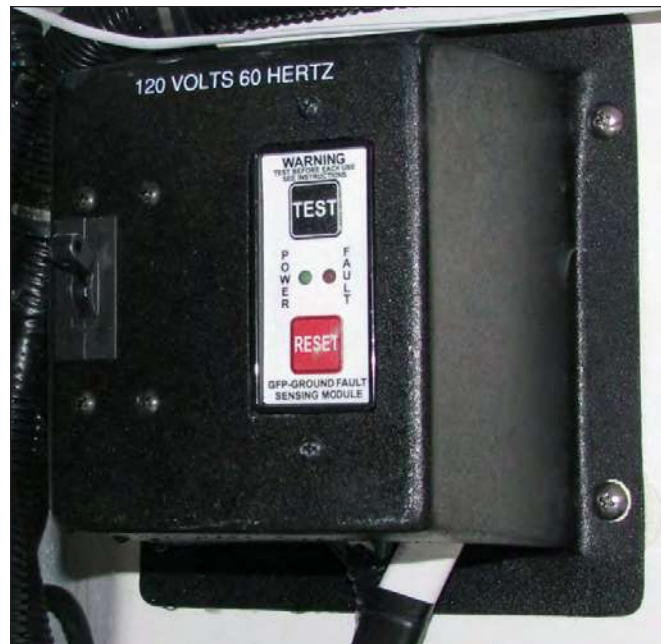
Typical Equipment Leakage Circuit Interrupter (ELCI) and Shore Main Inlet Breaker
