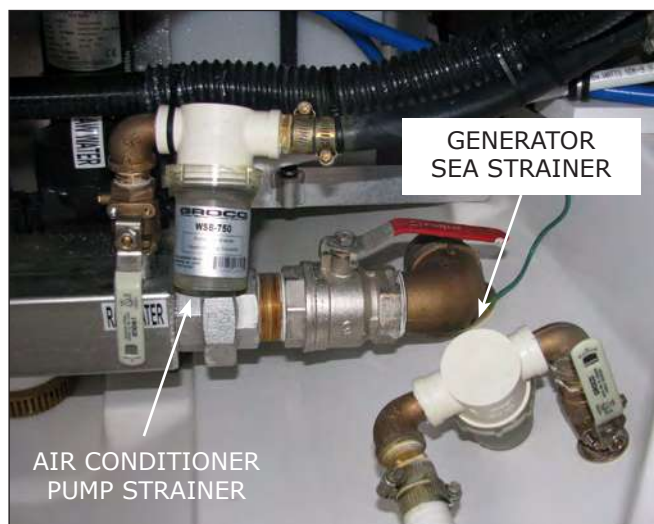
Air Conditioning Raw Water Strainer and Generator Cooling system Strainer
