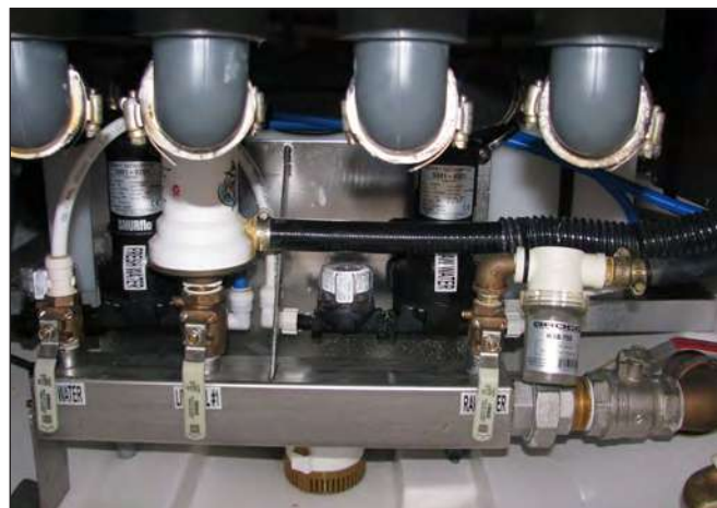
Raw Water Manifold, Baitwell Pump, Raw Water Supply Pump Connections and Ball Valves
