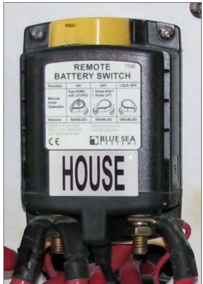
Typical Remote Battery Switch
