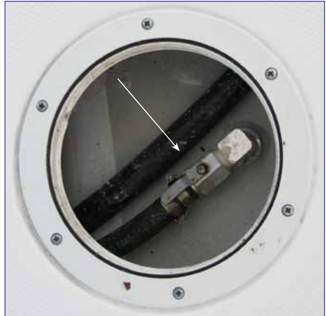
Typical Fuel Shutoff Valve
