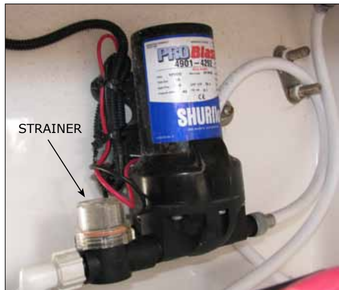
Typical Fresh Water Pump and Strainer
