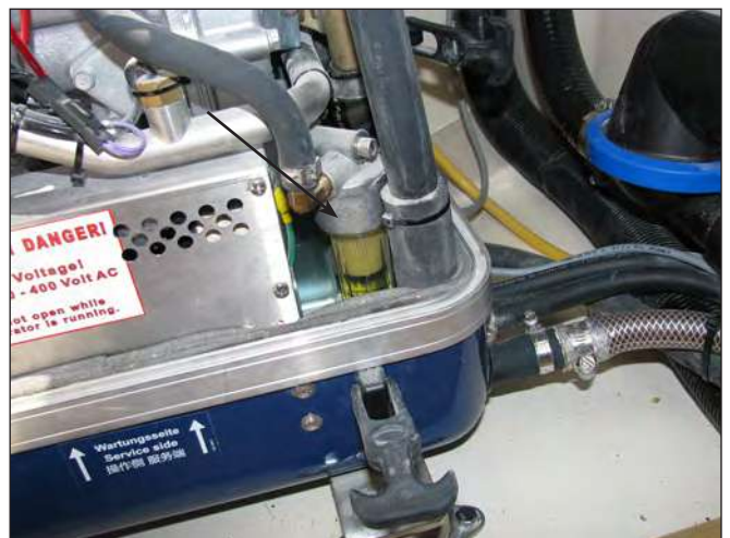
Typical Fuel Filter On the Generator
