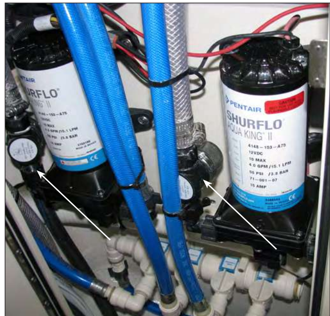
Typical Fresh Water Pump Strainers
