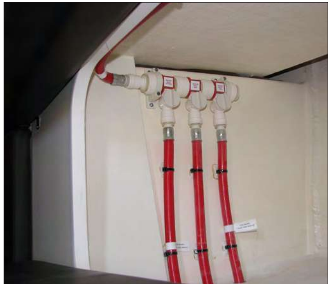
Hot Water Shutoff Valves Near Water Tank
