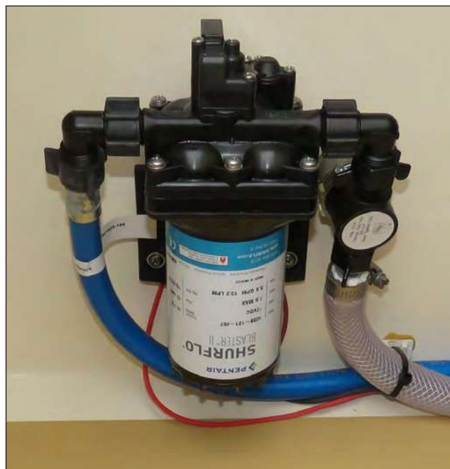
Typical Fresh Water Pump & Strainer
