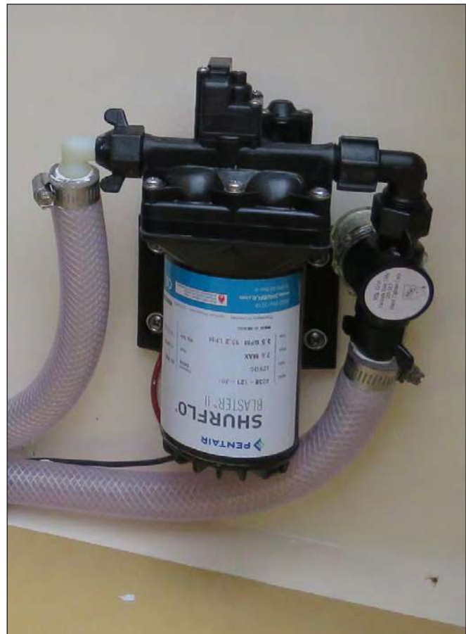
Raw Water Washdown Pump & Strainer
