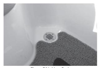
Figure B31: Liner Drain
