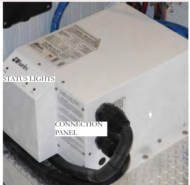
ISO BOOST ISOLATION TRANSFORMER
