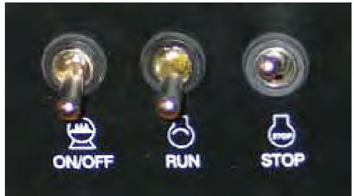
TYPICAL GEN-SET SWITCH CLUSTER- MAIN PANEL
