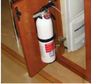
Typical Portable Fire Extinguisher
