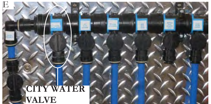
E CITY WATER VALVE FRESH WATER MANIFOLD-ENGINE ROOM
