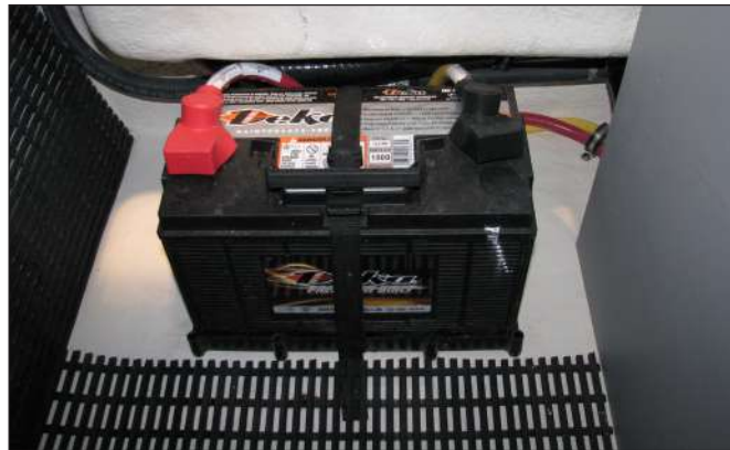
268SS Battery Installation
