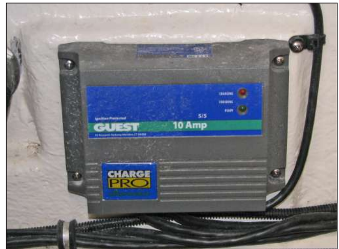
Typical Battery Charger
