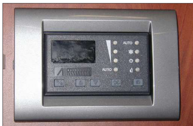
Typical Air Conditioner Control Panel
