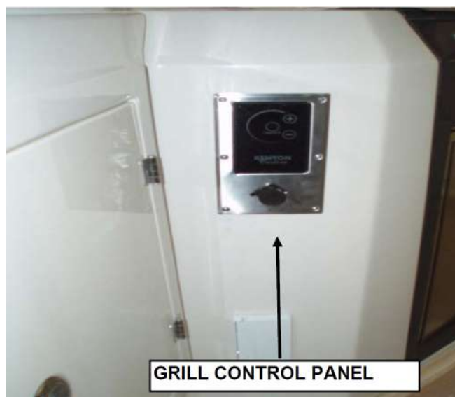
328SS Remote Grill Control Panel Near Battery Switch Panel In Cockpit
