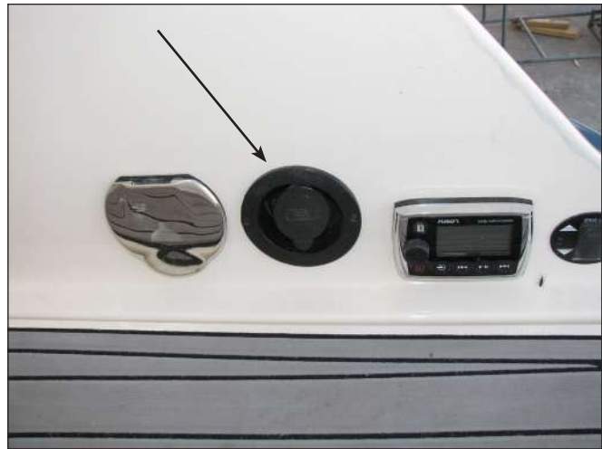
AC Battery Charger System Inlet Connection
