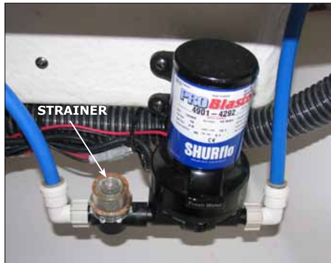
Typical Fresh Water Pump and Strainer
